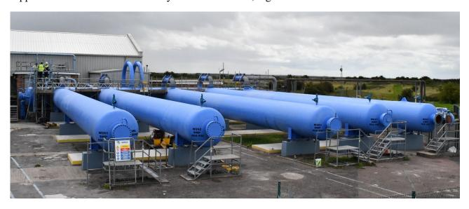
FCL formulated a staged approach to assessing the integrity of the units, with an initial phase of work aimed at providing confidence that the vessels remained safe for a limited period of further operation at somewhat reduced capacity, sufficient to enable continued use of the plant while more detailed fatigue assessment could be performed with the aim of justifying a longer period of future operation.
