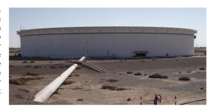
This was achieved by mechanical design substantiation of the new nozzles against the requirements of BS 2654 and relevant client standards, together with an assessment of critical defect sizes at selected weld locations at and adjacent to the new nozzles which was carried out in accordance with BS 7910.
